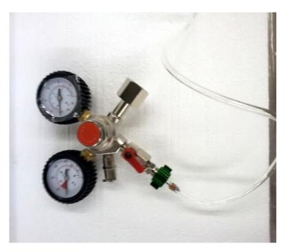
**Step 4: Attach Co2 Regulator to Co2 Tank**
